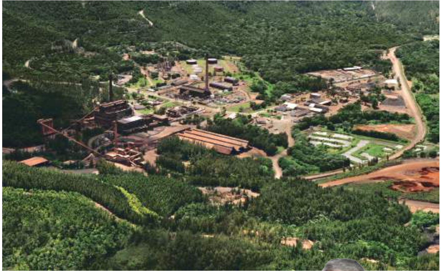
Aerial view of the Falcondo plant, Bonaó, Dominican Republic.
