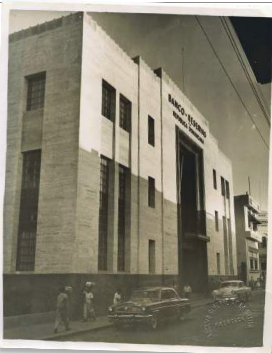
SANTO DOMINGO 1956 | Panoramic view of the Banco de Reservas de la República Dominicana Headquarters Building Opened in 1955 | Architect Alexander Aaron. Source: AGN. imágenes de nuestra historia ®.
